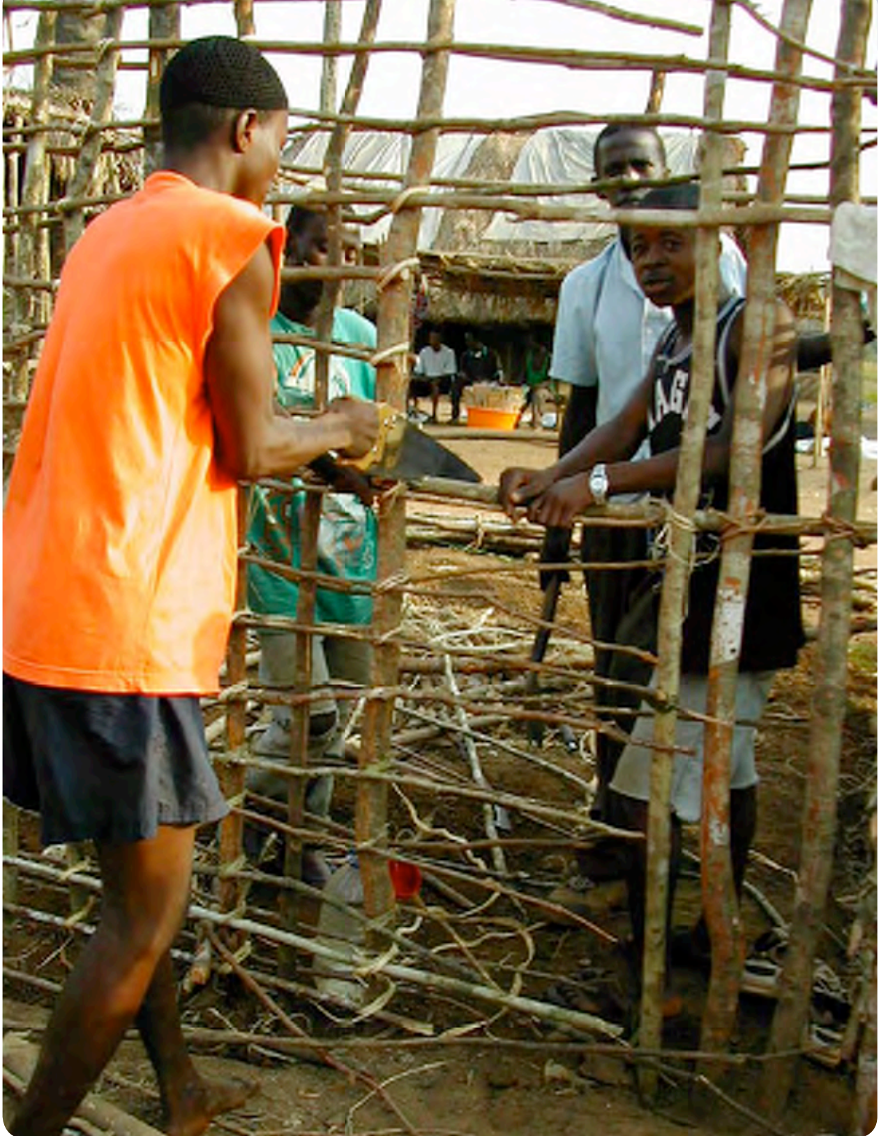
Newly arrived Liberian refugees in Jembe Camp in Sierra Leone help each other construct their new houses. Photo: Eduard Compte Verdaguer
